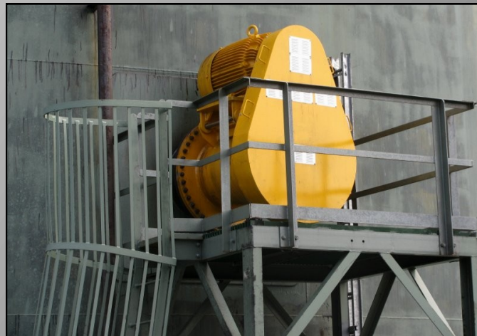
Above: A JM Engineering belt drive side entry mixer reducing sludge build up in a large petrochemical storage facility.
